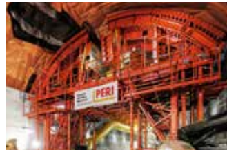
Tunnel Formwork
