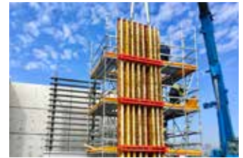
Column Formwork
