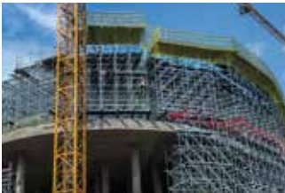
Beam and Slab Support
